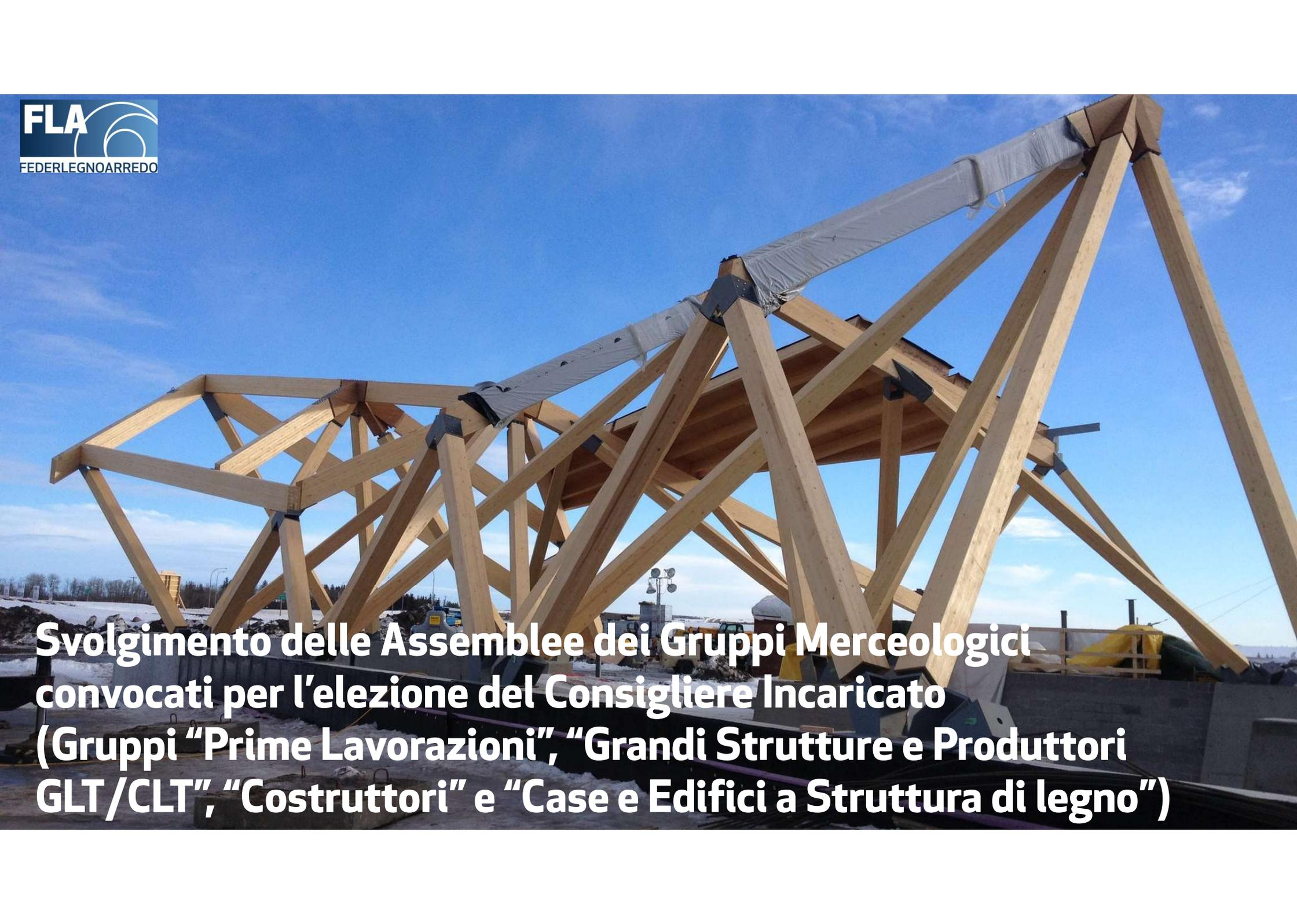
A large-scale construction site featuring a complex wooden truss structure. The structure is composed of numerous light-colored wooden beams, including vertical posts, horizontal beams, and diagonal bracing, all interconnected with metal brackets and bolts. The structure is set against a clear blue sky with a few wispy clouds. In the background, there are some construction materials, a yellow crane, and a building under construction. The ground appears to be a mix of dirt and snow.
